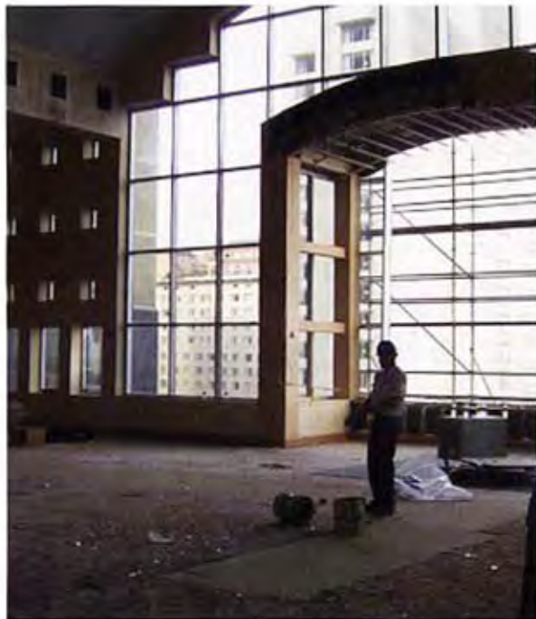
The Sheraton New Orleans' damaged ballroom being renovated by Montgomery Roth.
