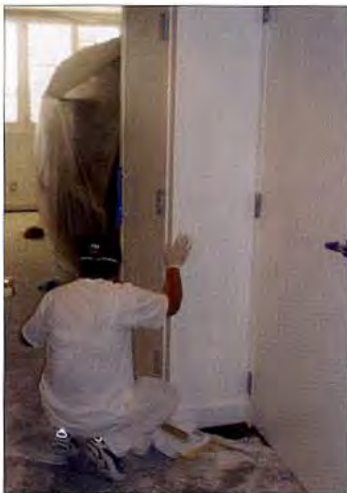
Workers paint the hallways of the W New Orleans.
